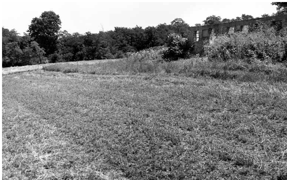
Fig. 1 Mekote locality and walls of abandoned stable in Nemenikuće
